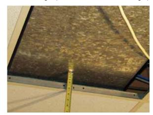
Drill 5 inch hole in ceiling tiles or sheetrock. Supply 16 or 18 gauge 2 conductor wire for lights.
